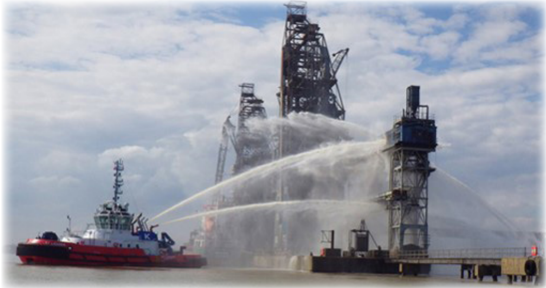
Image 1: Conveyor fire being extinguished
