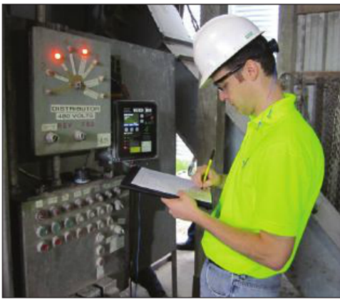
Brian Knapp, 4B Components vice president of technical sales and service-Electronics Division, performing a Tech Team inspection on a Watchdog Super Elite monitoring system.
