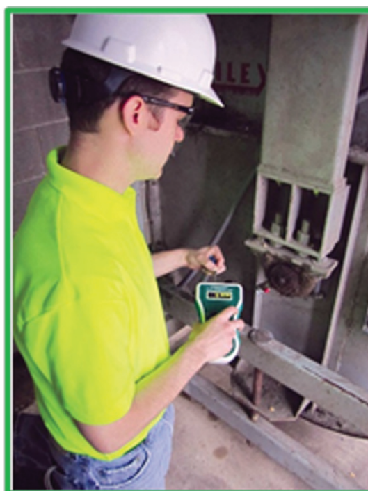
Bearing temperature sensor testing
