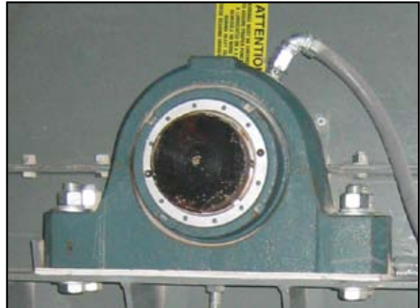
WDB20V3C bearing temperature sensor shown installed on a head bearing of a bucket elevator.
