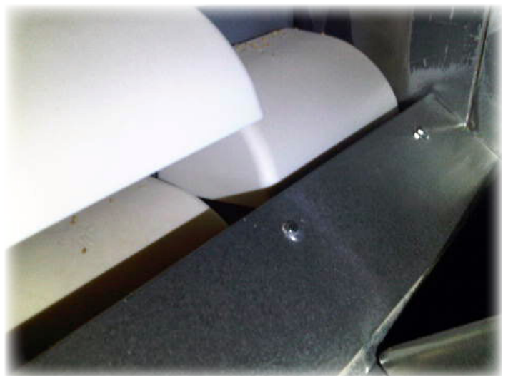
Image 5: SPS buckets installed
